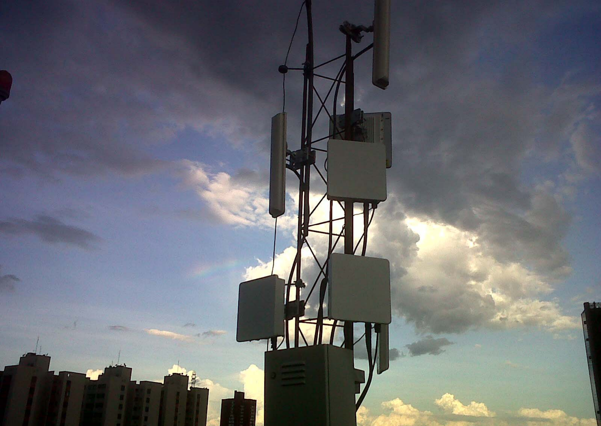
Tsunami Radios Backhauling Video Data to Central Monitoring Station
